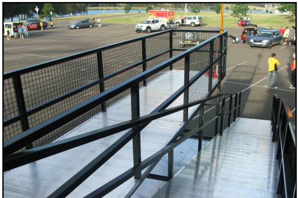
View from the top down the ramp.
